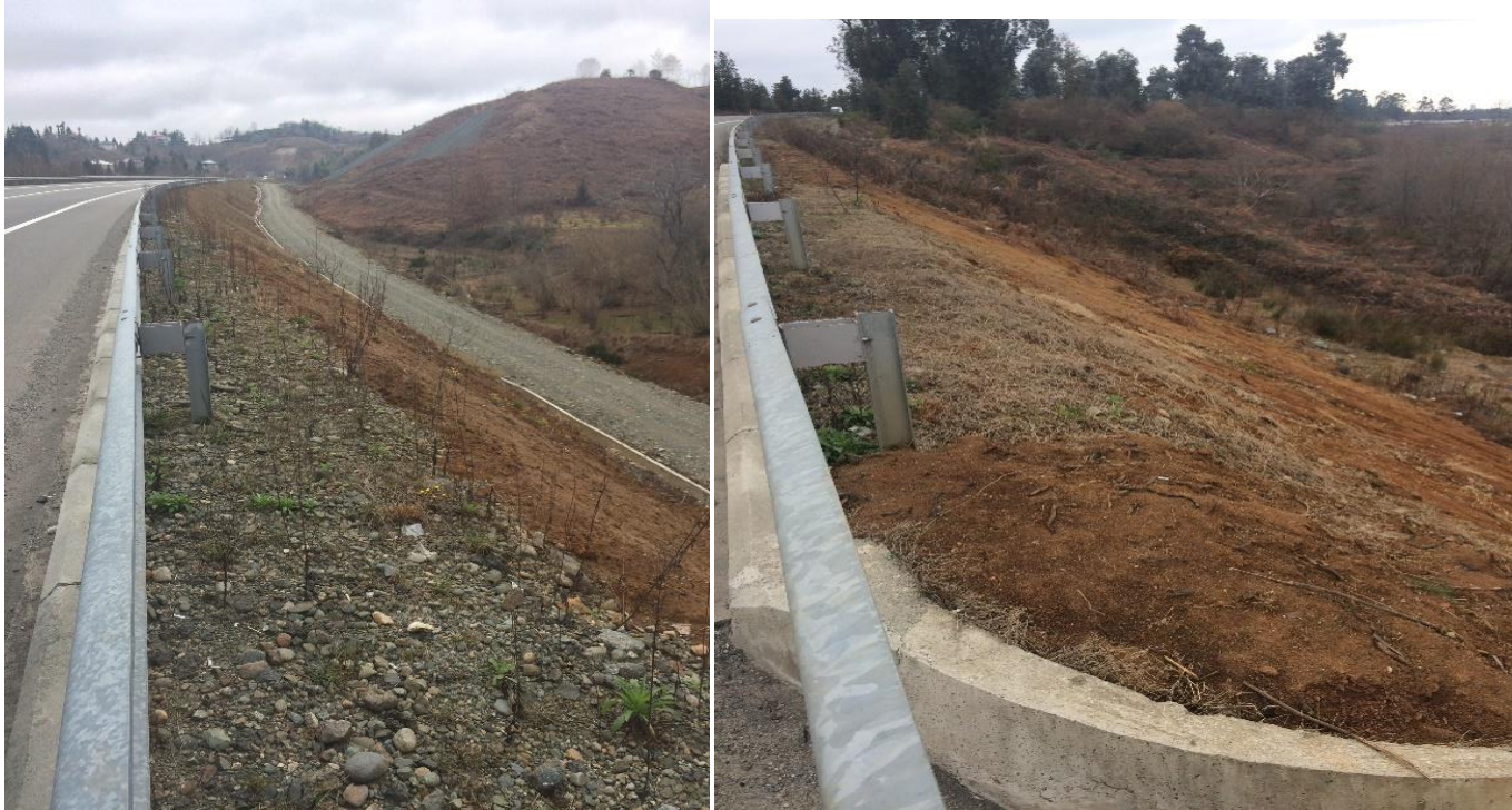
Photo 3. Slopes stabilization/reinstatement (KP 5 and KP 11,800)
